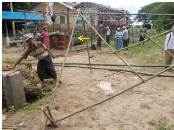
side rope (arrowed) being replaced by bamboo
