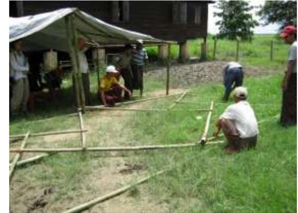
Laying out the two additional roof frames to mark the position of the support posts
