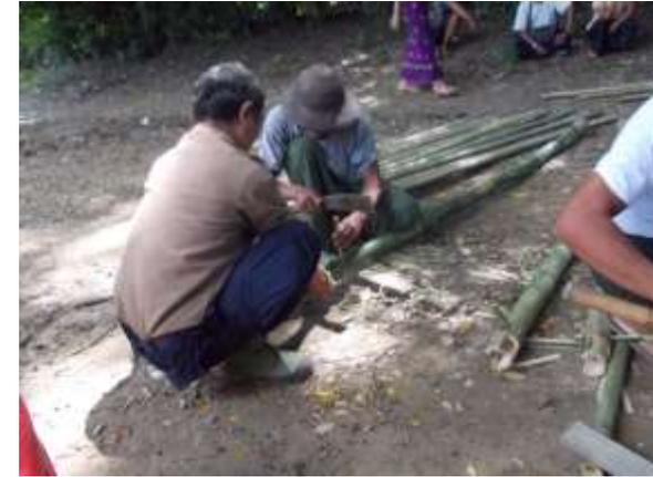
Cutting the dowel holes on the posts
