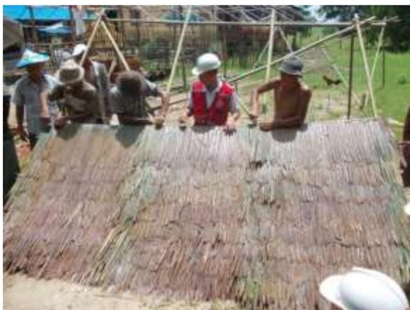
Frame support was remarkably flat with a good incline for water runoff
