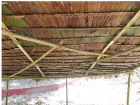
Loading is reasonably spread over the central frame. A third split bamboo pole lashed across the upper and lower intersecting frame points may be even better.
