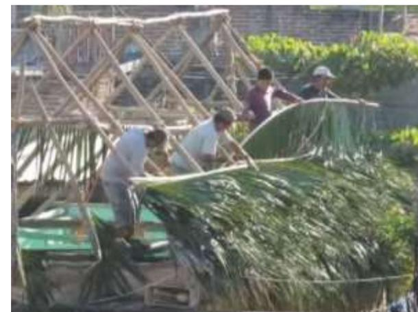
In an emergency split palm leaves, as used for thatching this permanent roof, would be layered from bottom to top.
