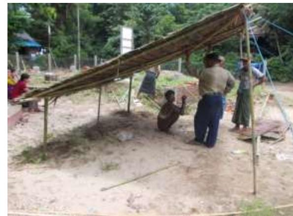
Shelter roof elevated. An additional central support has been added to the lower ridge pole.
